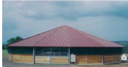
Spanish Riding School, Vienna, Austria, Ceiling Mounted Walker with metal roof and wind net
