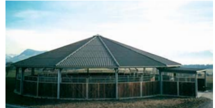
Paul Estermann Riding Sport Center, Hildisrieden, Switzerland, Ceiling Mounted Walker with corrugated cement fiber roof
